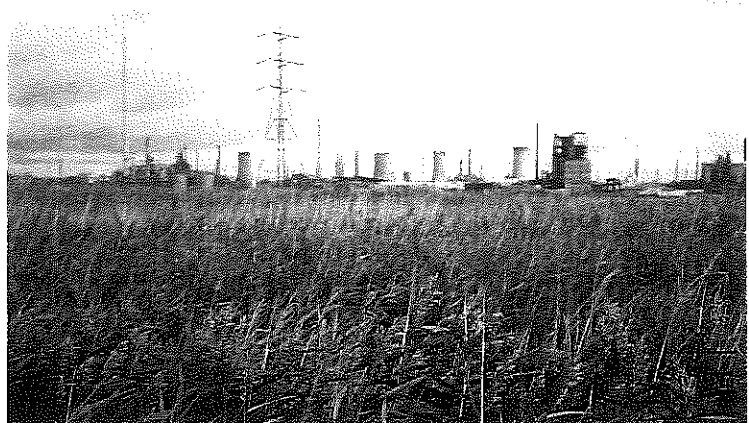
❖ Figure 22 Chemical waste from an industrial complex is being treated using reed beds. Bacteria and fungi in the reed beds transform a wide range of pollutants into harmless substances.
